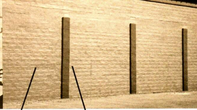
AFTER 4 YEARS, NO SIGN OF DETERIORATION OR MOISTURE PENETRATION.
